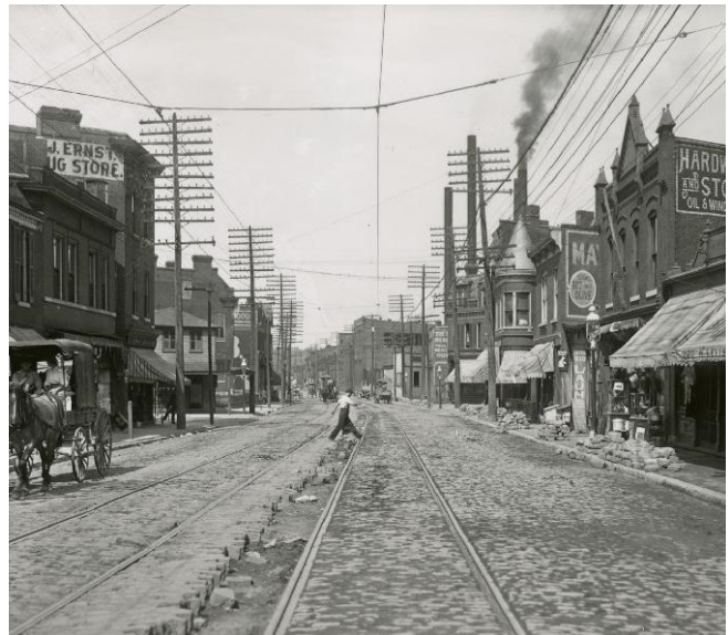
900 Block of Vandeventer with stones, 1921-1923.
